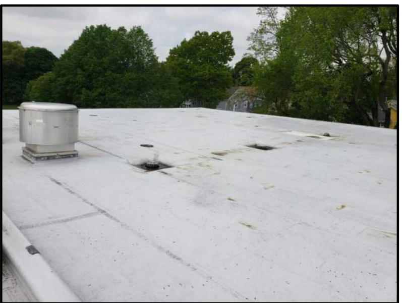
ROOF DRAINS ON 1955 ADDITION NO SCALE
