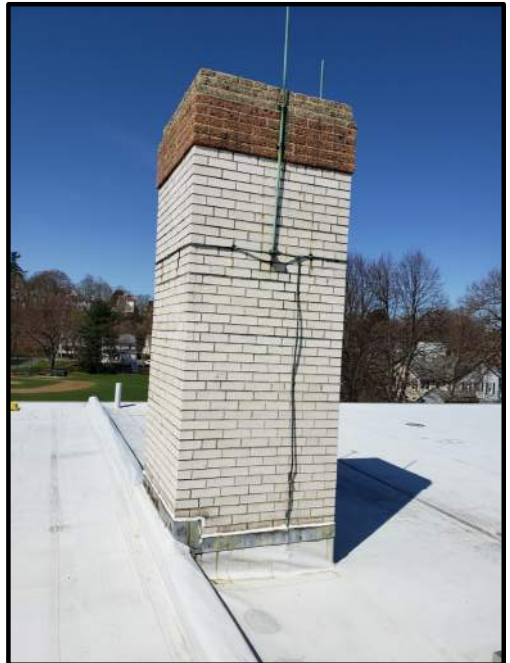
EXISTING CHIMNEY NO SCALE
