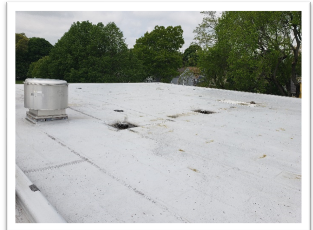
Photo 2: Existing Roof over 1955 Addition
