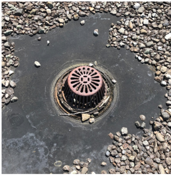
Photo 3: Roof Drain
