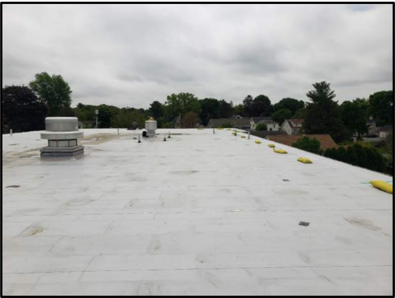
EXISTING ROOF OVER 1949 BUILDING NO SCALE
