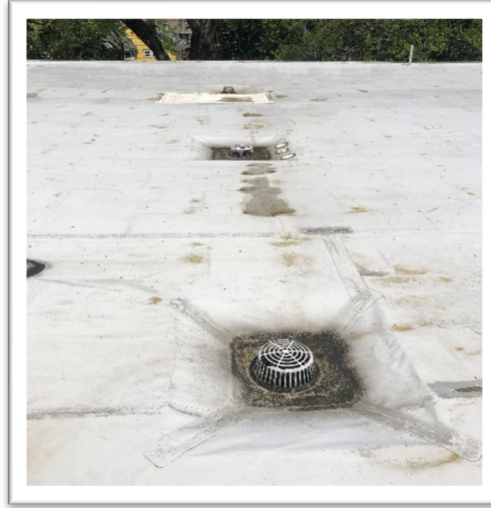
Photo 3: Existing Roof Drains
