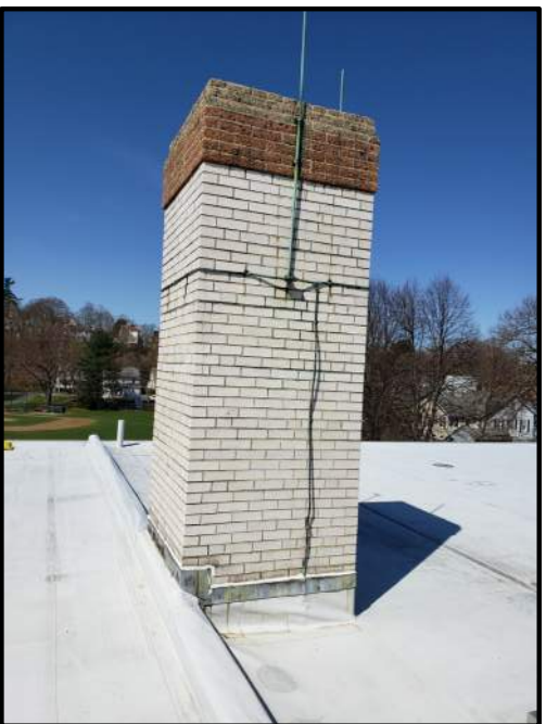
EXISTING CHIMNEY NO SCALE
