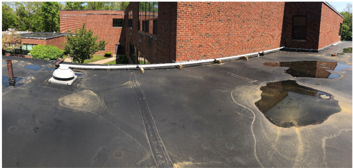
Photo 5: Storm Leader Routed on Roof
