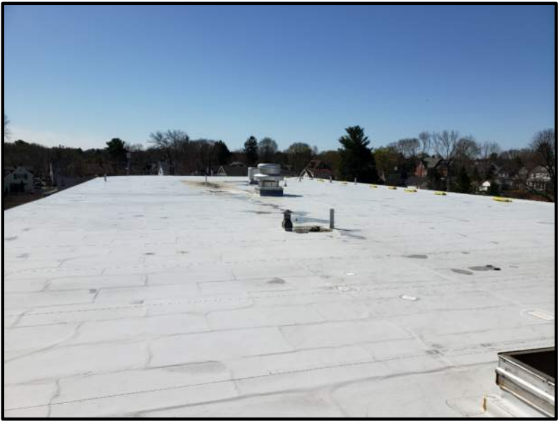
EXISTING ROOF OVER 1949 BUILDING NO SCALE
