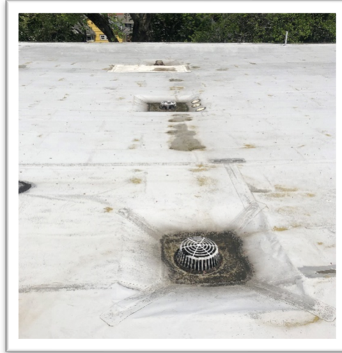
Photo 3: Existing Roof Drains
