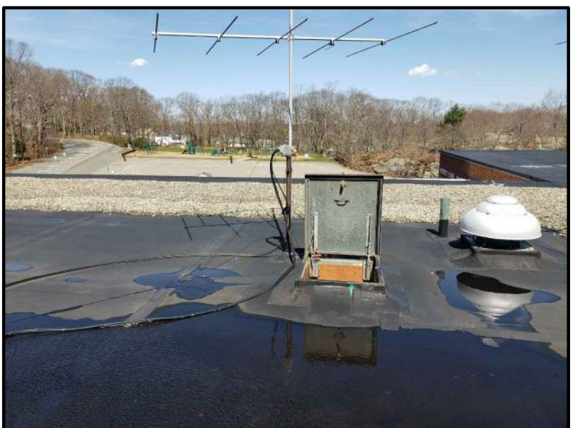
ROOF ACCESS HATCH NO SCALE D -
