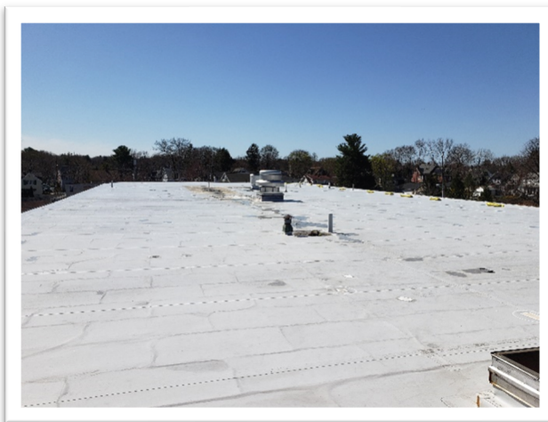
Photo 1: Existing Roof over 1949 Building
