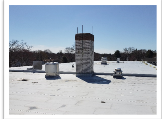
Photo 5: Equipment and Chimney on 1955 Building Addition
