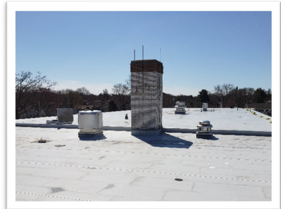
Photo 5: Equipment and Chimney on 1955 Building Addition
