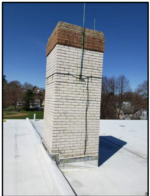
EXISTING CHIMNEY NO SCALE
