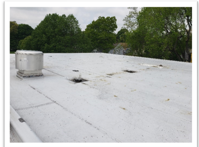
Photo 2: Existing Roof over 1955 Addition
