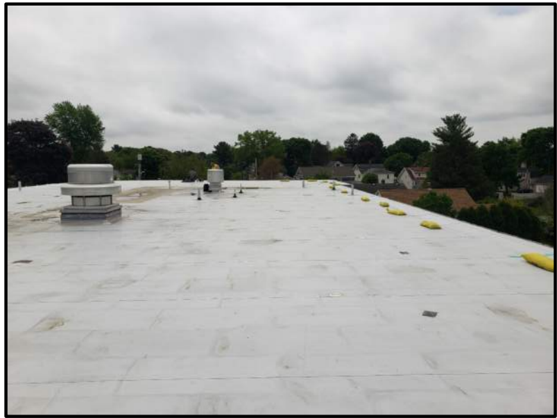
EXISTING ROOF OVER 1949 BUILDING NO SCALE
