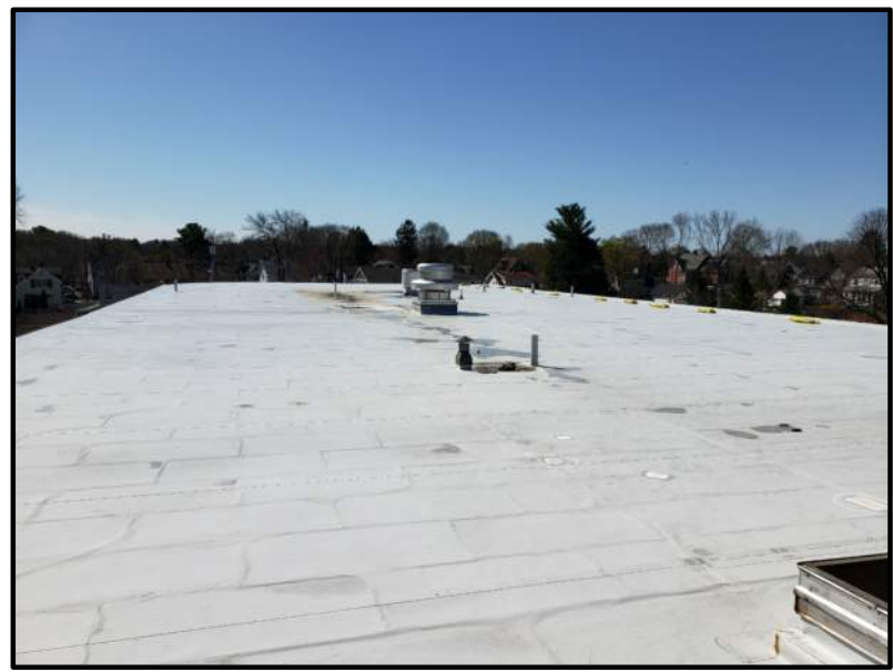
EXISTING ROOF OVER 1949 BUILDING NO SCALE
