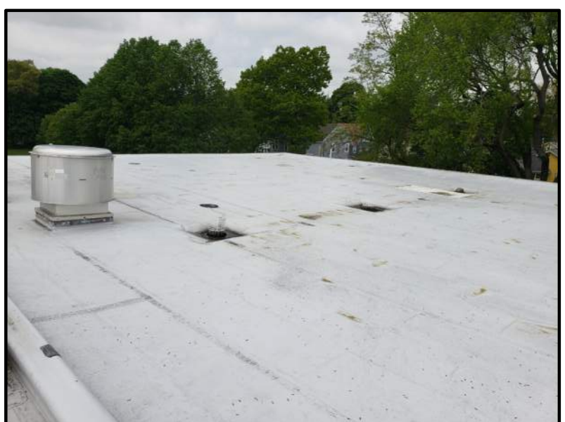
ROOF DRAINS ON 1955 ADDITION NO SCALE
