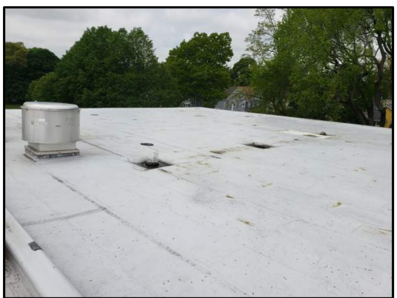
ROOF DRAINS ON 1955 ADDITION NO SCALE
