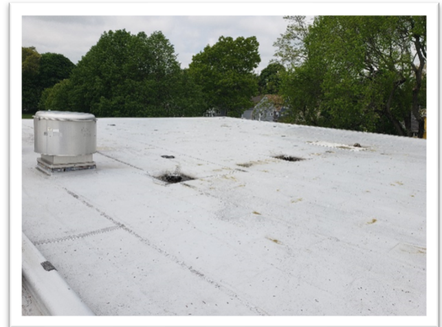
Photo 2: Existing Roof over 1955 Addition
