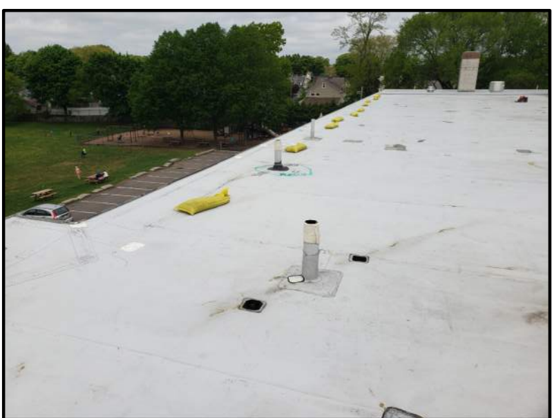
EXISTING VENT PENETRATIONS NO SCALE
