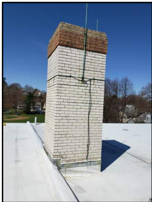
EXISTING CHIMNEY NO SCALE
