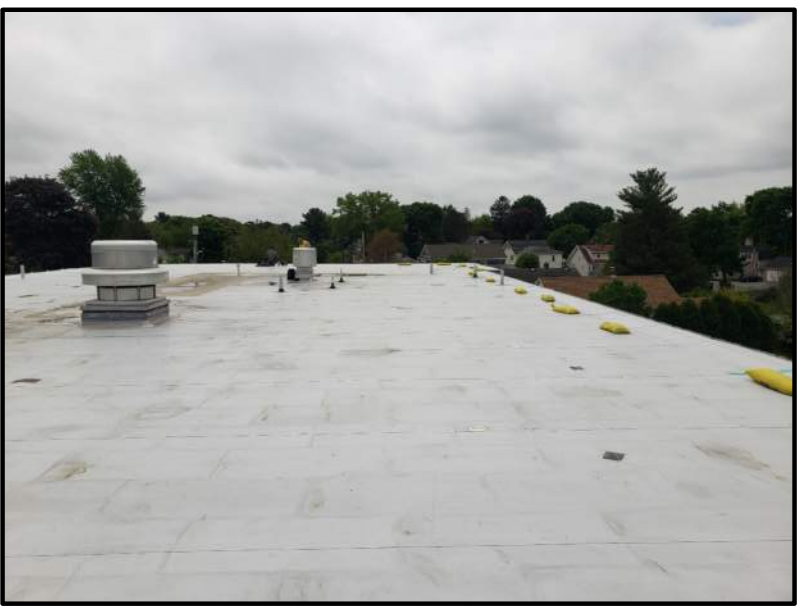
EXISTING ROOF OVER 1949 BUILDING NO SCALE
