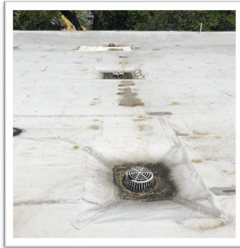
Photo 3: Existing Roof Drains
