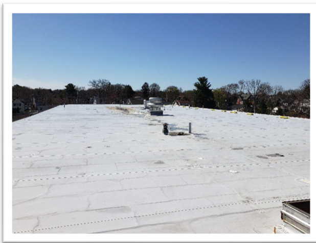
Photo 1: Existing Roof over 1949 Building
