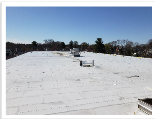
Photo 1: Existing Roof over 1949 Building
