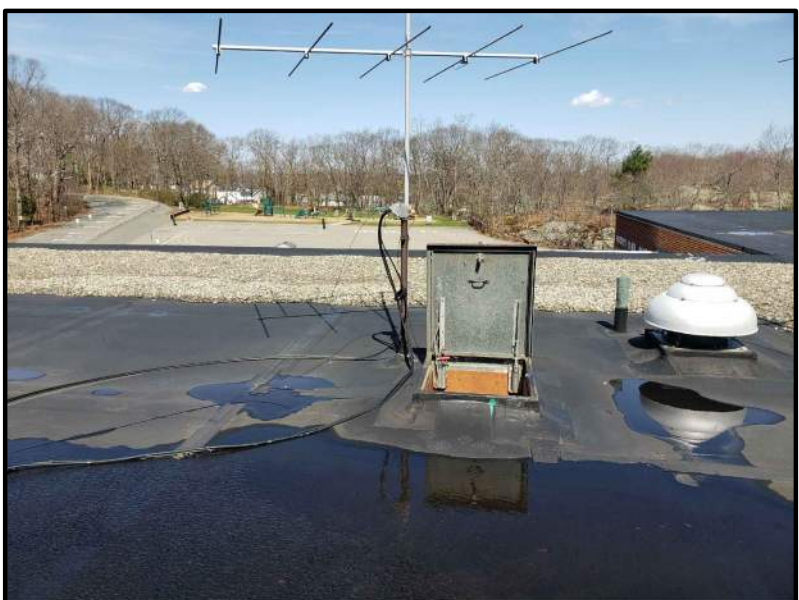
ROOF ACCESS HATCH NO SCALE D -
