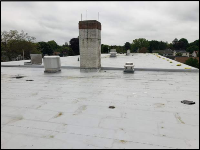
CHIMNEY AND EQUIPMENT ON 1955 ADDITION NO SCALE
