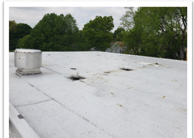
Photo 2: Existing Roof over 1955 Addition
