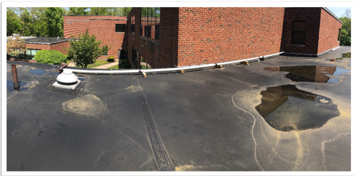
Photo 5: Storm Leader Routed on Roof
