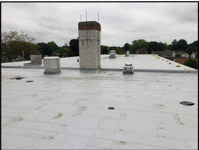
CHIMNEY AND EQUIPMENT ON 1955 ADDITION NO SCALE
