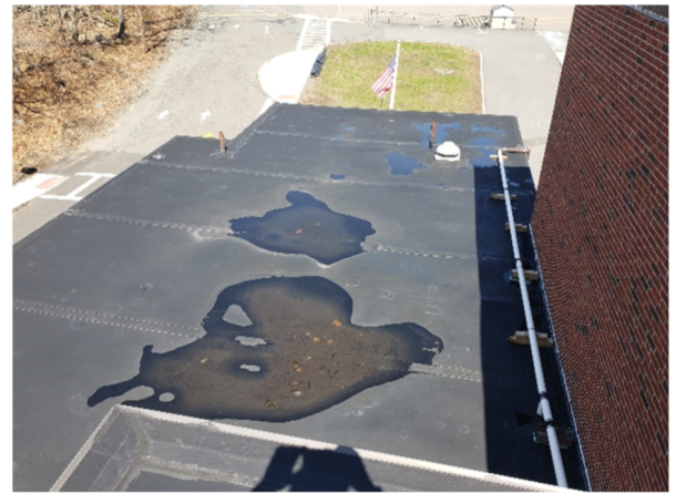
Photo 2: Roof Over Lower Building
