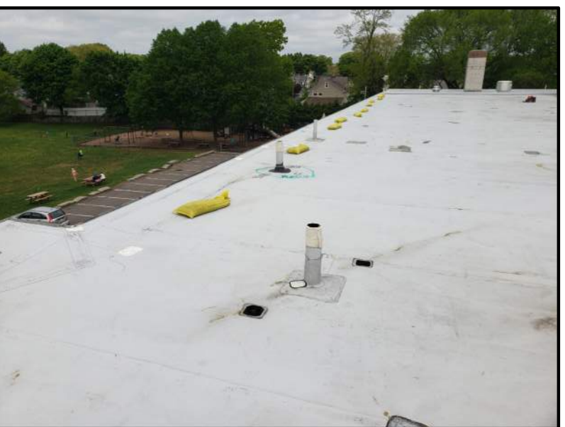
EXISTING VENT PENETRATIONS NO SCALE
