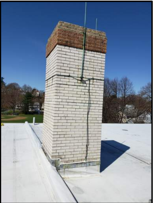
EXISTING CHIMNEY NO SCALE
