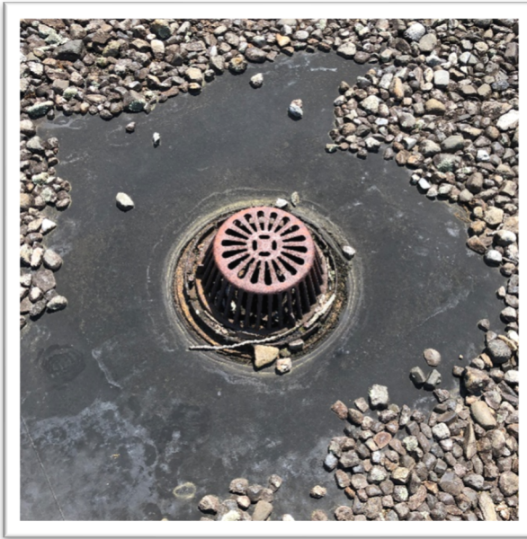
Photo 3: Roof Drain
