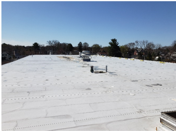
Photo 1: Existing Roof over 1949 Building
