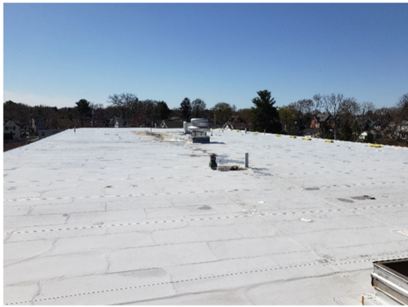
Photo 1: Existing Roof over 1949 Building
