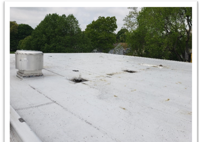
Photo 2: Existing Roof over 1955 Addition
