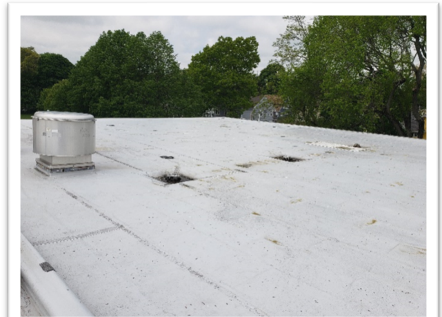
Photo 2: Existing Roof over 1955 Addition
