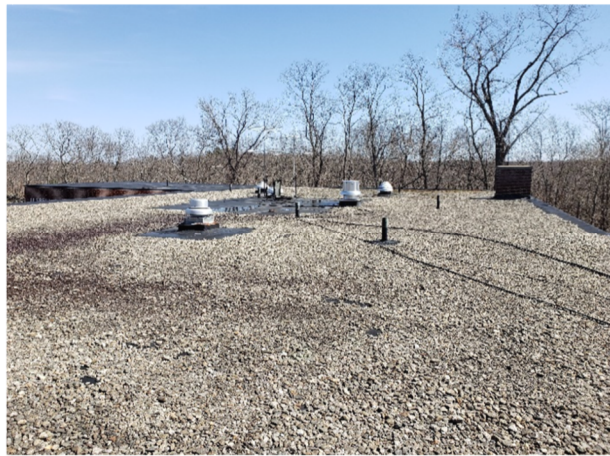
Photo 1: Roof Over Main Building
