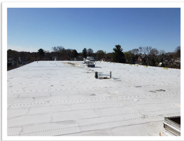
Photo 1: Existing Roof over 1949 Building
