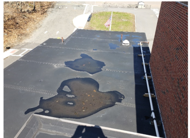
Photo 2: Roof Over Lower Building
