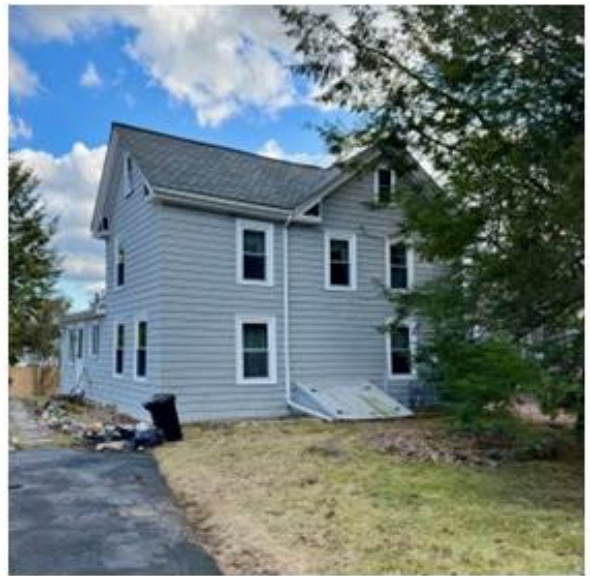
Rear of the Jabez Lynde / Grundy House
