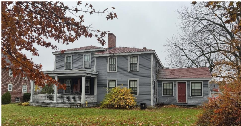
East Facades facing Main Street- 2025 photo by Rob Tullis, Melrose Hist. Dist. Comm.
