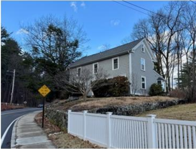
Jabez Lynde / Grundy House, c. 1700 407 Washington Street, adjacent to the Saugus town line
