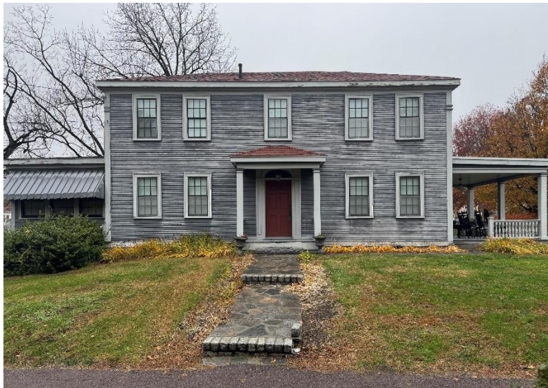
South /Front Facade- 2025 photo by Rob Tullis, Melrose Hist. Dist. Comm.
