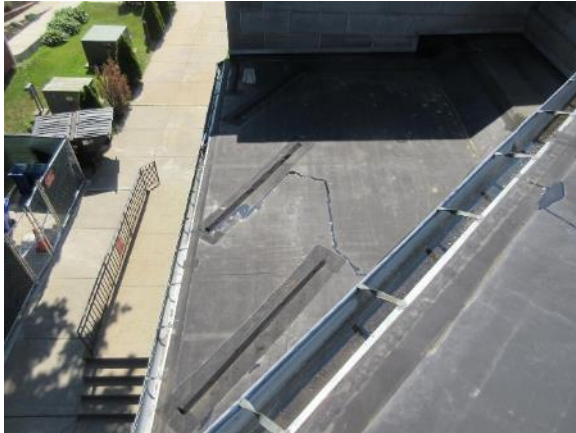
Image 91: Rain diverters installed on Roof Area F
