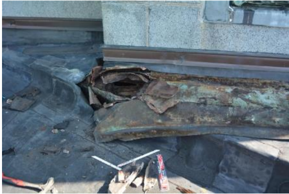
Image 11: Location of steel exploration at Roof Area E
