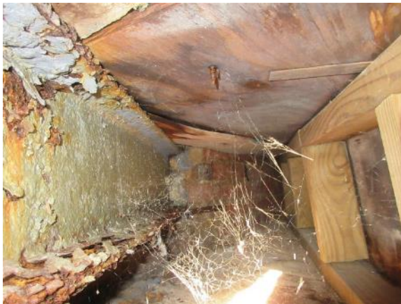
Image 11: View underneath the raised curb looking down along the diagonal member towards its embedment.
