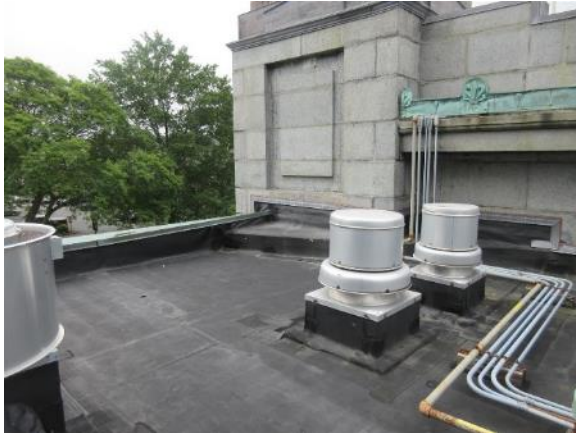
Image 87: Overall image of Roof Area C
