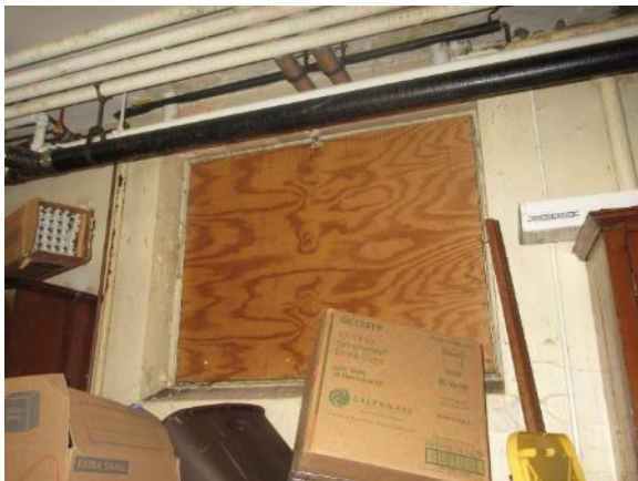
Image 49: Typical installation of a plywood blank-off panel on the interior; this image taken within the basement storage room at the northeast corner of the building.
