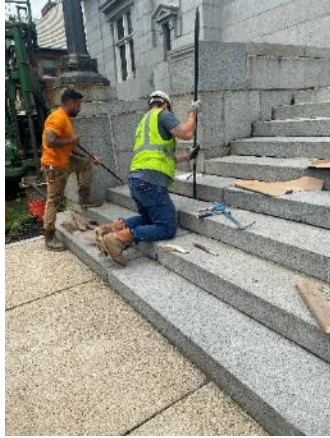
Image 119: Location of stair removal
