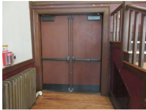
Image 72: Typical interior of the auditorium side doors (Door 103)
