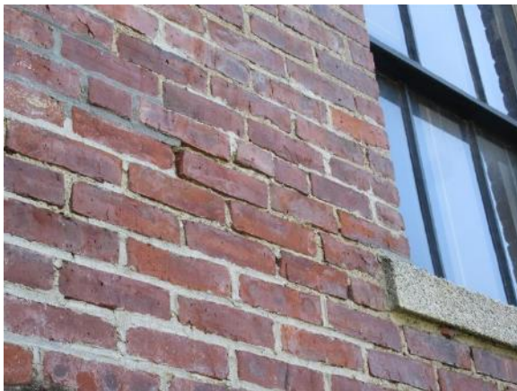
Image 23: Typical mortar condition within the brick masonry at the Addition
