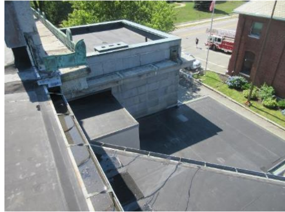
Image 88: Overall image of Roof Areas E, G, and H
