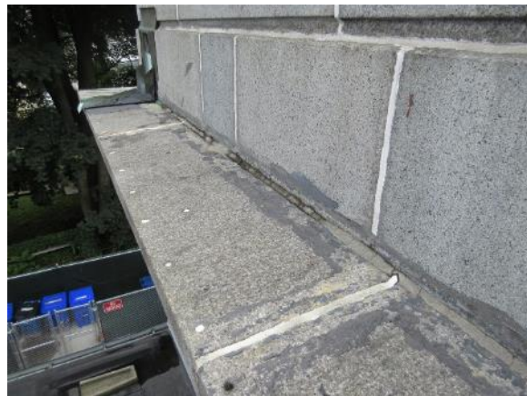
Image 20: Sealant repairs at the granite ledge on the west side of the North Wing
