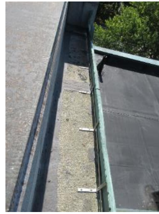
Image 34: Typical horizontal banding attachment straps.
