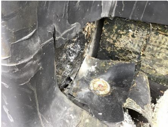
Image 99: A gap in the granite wall was observed at Test Cut #13.
