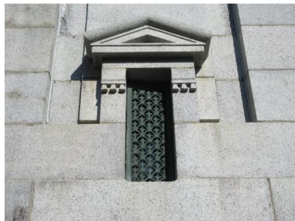
Image 38: Typical brass grille installed over small windows on the Front (East) Elevation.
