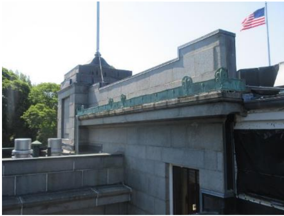
Image 33: Horizontal brass banding at Roof Area A parapet ledge on the North Elevation.
