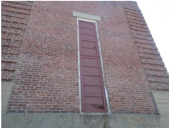
Image 75: Exterior of the organ access door.
