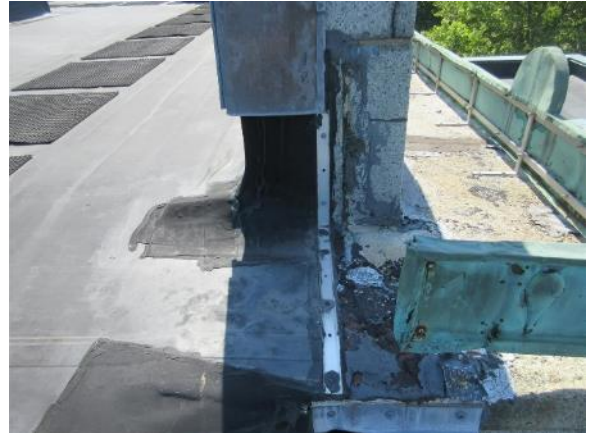
Image 104: Membrane terminated with an exposed termination bar at the transition to the granite ledges on Roof Area A.
