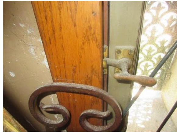
Image 58: Typical hand and lock hardware at swinging casement windows.
