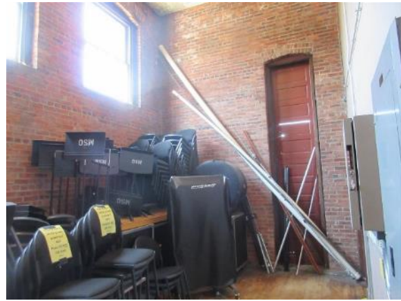
Image 76: Interior of the organ access door.
