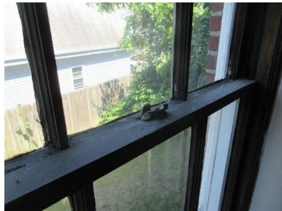
Image 56: Typical brass lock hardware at hung windows.
