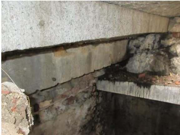
Image 121: View within the cavity looking towards the front of the stair. The foundation was found to be a combination of concrete stem walls, brick masonry, granite slabs, and rubble.
