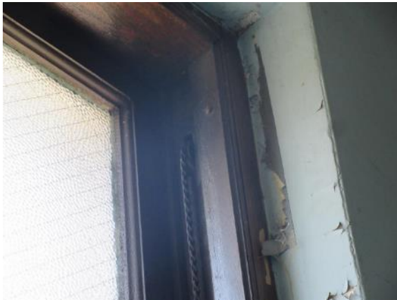
Image 57: Typical chain and pulley hardware at hung windows.
