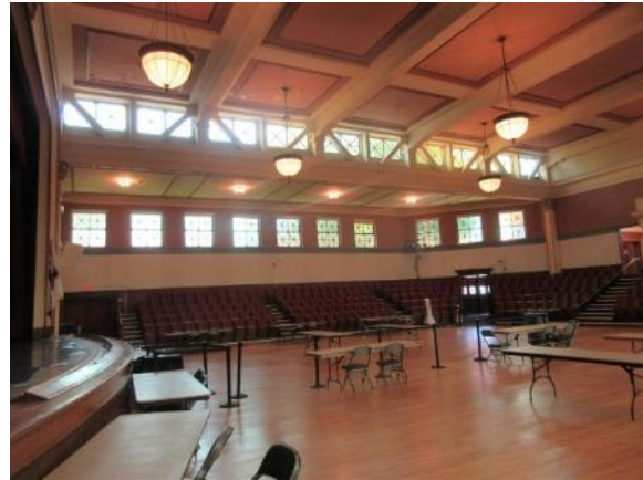
Image 46: View of the auditorium space with the bands of upper and lower clerestory windows.
