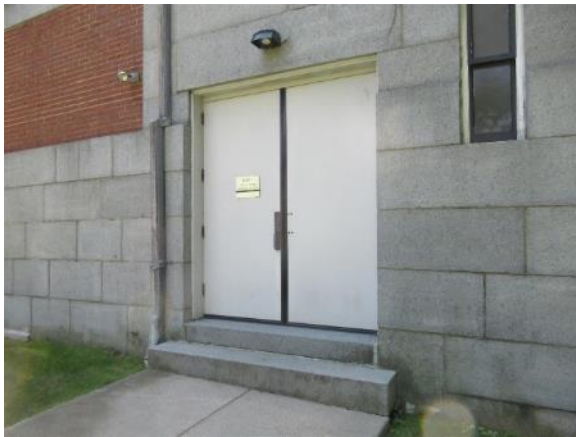
Image 71: Typical exterior of the auditorium side doors (Door 103)
