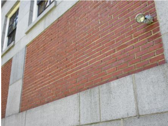
Image 25: Typical brick inset area at the original building
