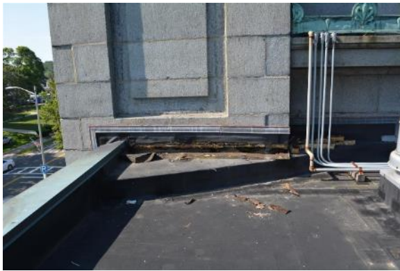
Image 11: Location of steel exploration at Roof Area D at the base of the flagpole rising wall
