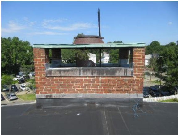
Image 113: Overall view of the chimney
