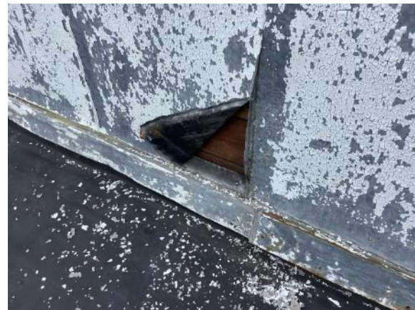
Image 102: A portion of the sheet metal siding was lifted open to reveal a wood back-up wall, which appeared to be in good condition.
