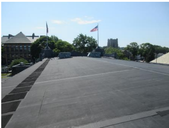
Image 85: Overall image of Roof Area A
