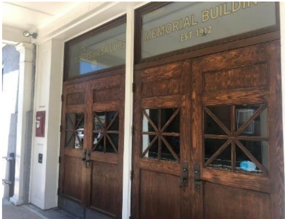
Image 79: Exterior of the main entrance doors.
