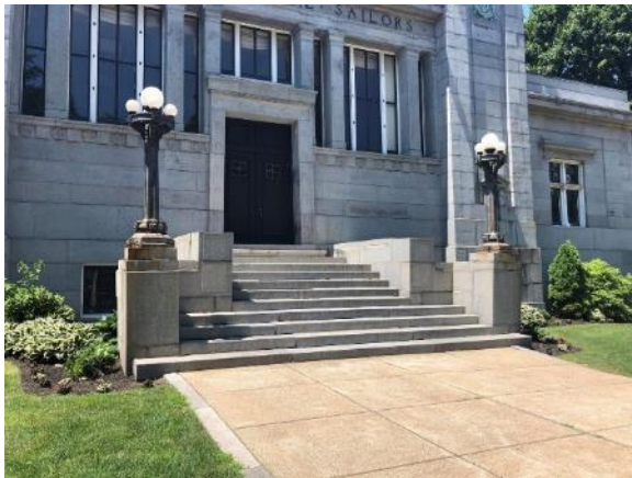
Image 117: Overall view of the front entrance stairs
