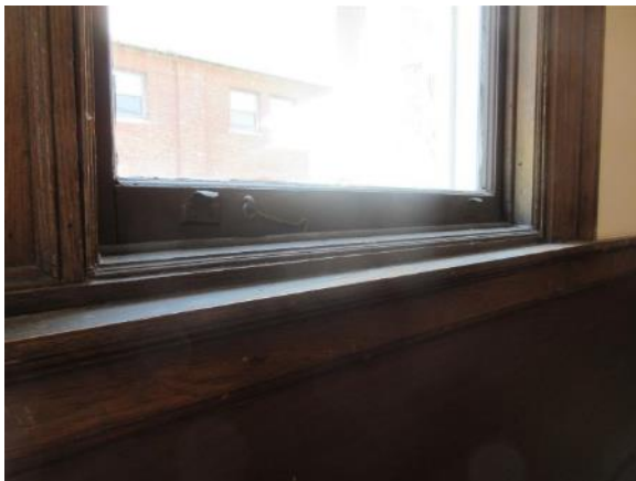
Image 55: Typical brass handles installed at Window Type D.
