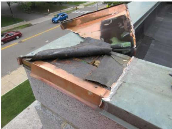
Image 101: Test Cut #15 was performed at the corner of Roof Area D to open the parapet cap
