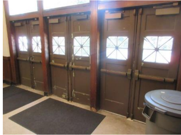
Image 66: Interior of the south lobby entrance doors
