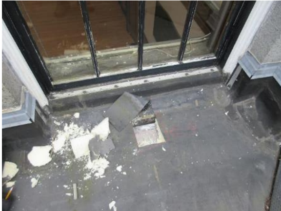
Image 97: Test Cut #8 performed at the sill of Window Type H. The roof membrane was found to be terminated on the window sill with a termination bar.
