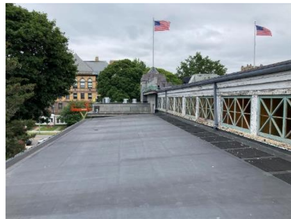
Image 86: Overall image of Roof Area B
