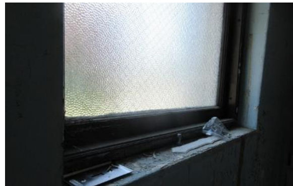
Image 54: Typical obscured glazing within bathrooms and storage closets on the first floor.
